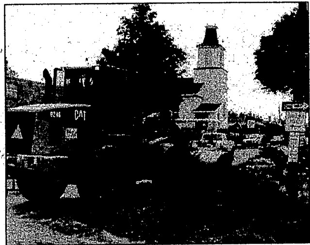
MDOT workers continue to work on Main Street Photo by Ed Davis
