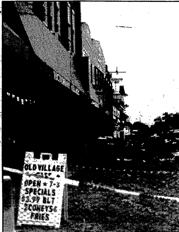
Under construction--Main Street undergoes improvements. File photo.
