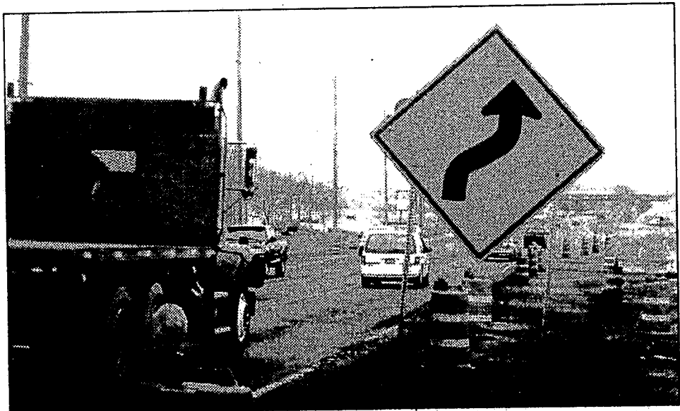
Motorists on Dixie Highway between I-75 and Davisburg Road will have to navigate a three-lane highway until April 2003, when plans to widen Dixie to five lanes will resume. Photo by Jeff Patrus.
