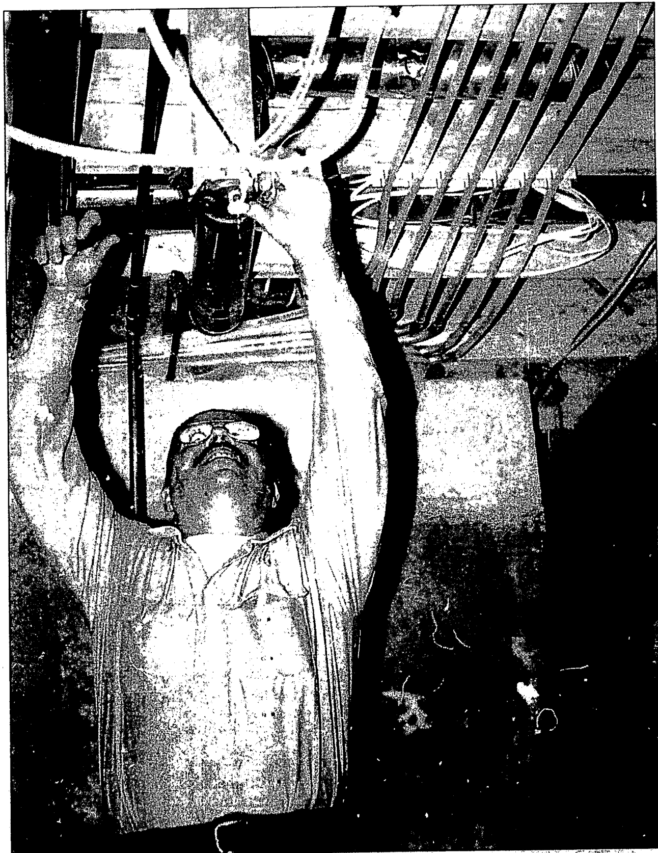
Plumber John Muse works on a sprinkler head for the new Wirsbo multipurpose fire suppression system, a plumbing/sprinkler system for single-family homes. The first home in Michigan to have the system installed is located in Independence Township. Photo by Jennifer Nemer.
