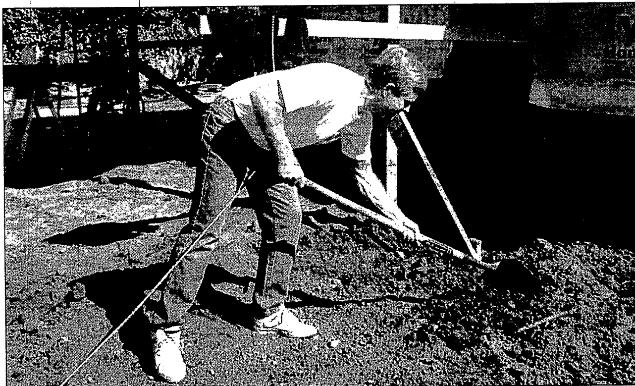
Pastor Greg Henneman of Clarkston Community Church shovels some dirt at the Habitat for Humanity home in Pontiac. Volunteers from Clarkston Community Church and St. Daniel Catholic Church in Clarkston helped put the home together. Photo provided.
