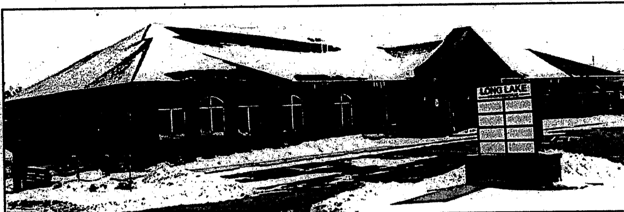
Oxford Bank's new Commercial Loan Center at 720 North Lapeer Road in Lake Orion.
