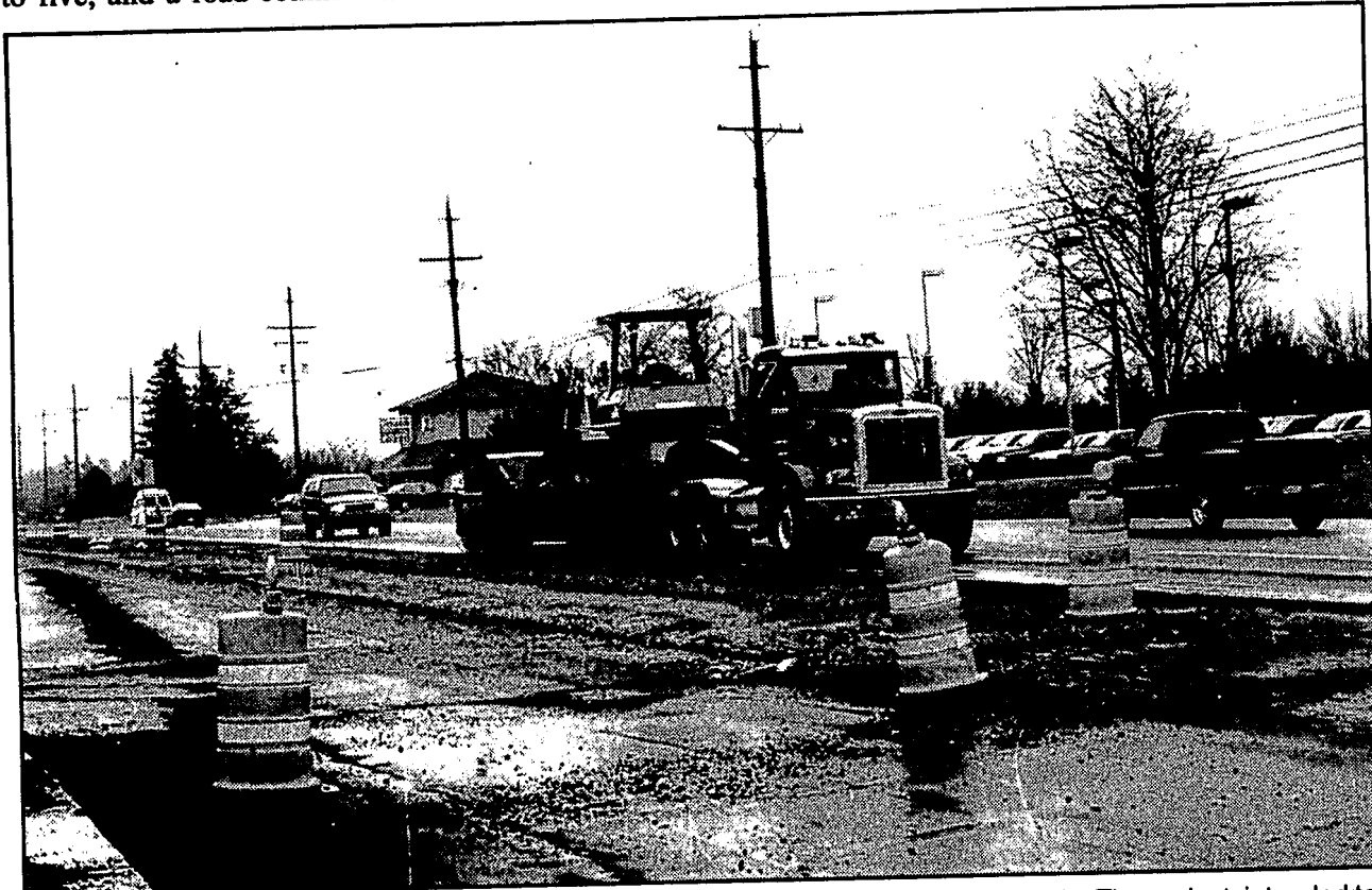
Traffic navigates past orange barrels on Dixie Highway near I-75 in Springfield Township. The project, intended to widen the roadway to five lanes to Davisburg Road, is scheduled to be complete by May 30. Photo by Don Schelske
