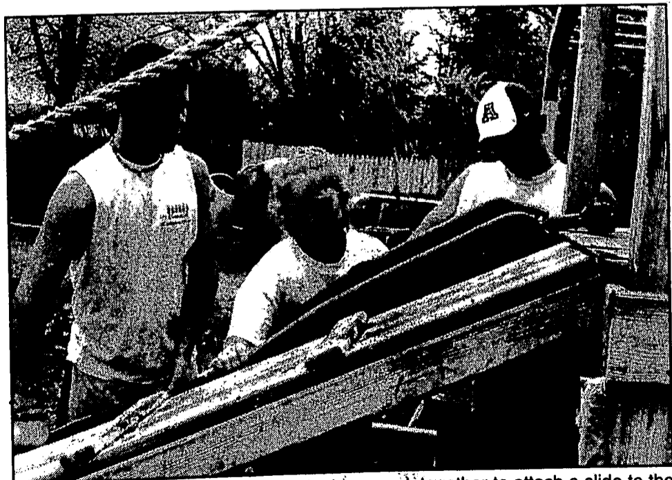
Ryan Kaltz, Kaitlin Kieras and Bob Andaray work together to attach a slide to the new swingset at the Andersonville Road home in Springfield Township.
