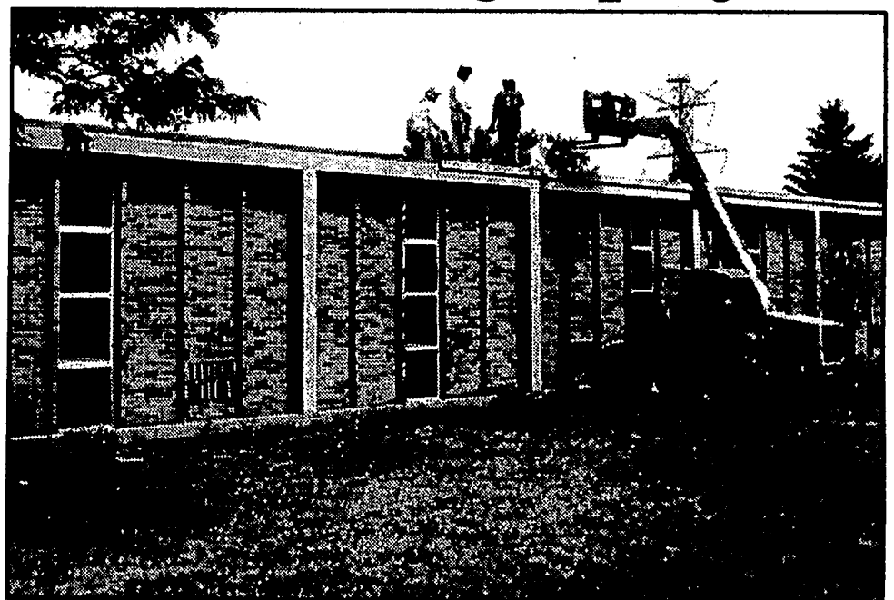
Workers load materials on the roof of Sashabaw Middle School, where work has begun on roof replacement. It is one of the first projects to be paid with money from the $83.7 million bond issue approved by voters June 9. Photo by Don Schelske
