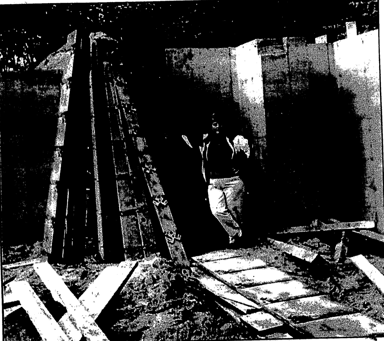
Sue Sajdak proudly stands on the construction site of her home, construction of which she supervised herself after earning her builder's license through Clarkston Community Education. Photo provided.
