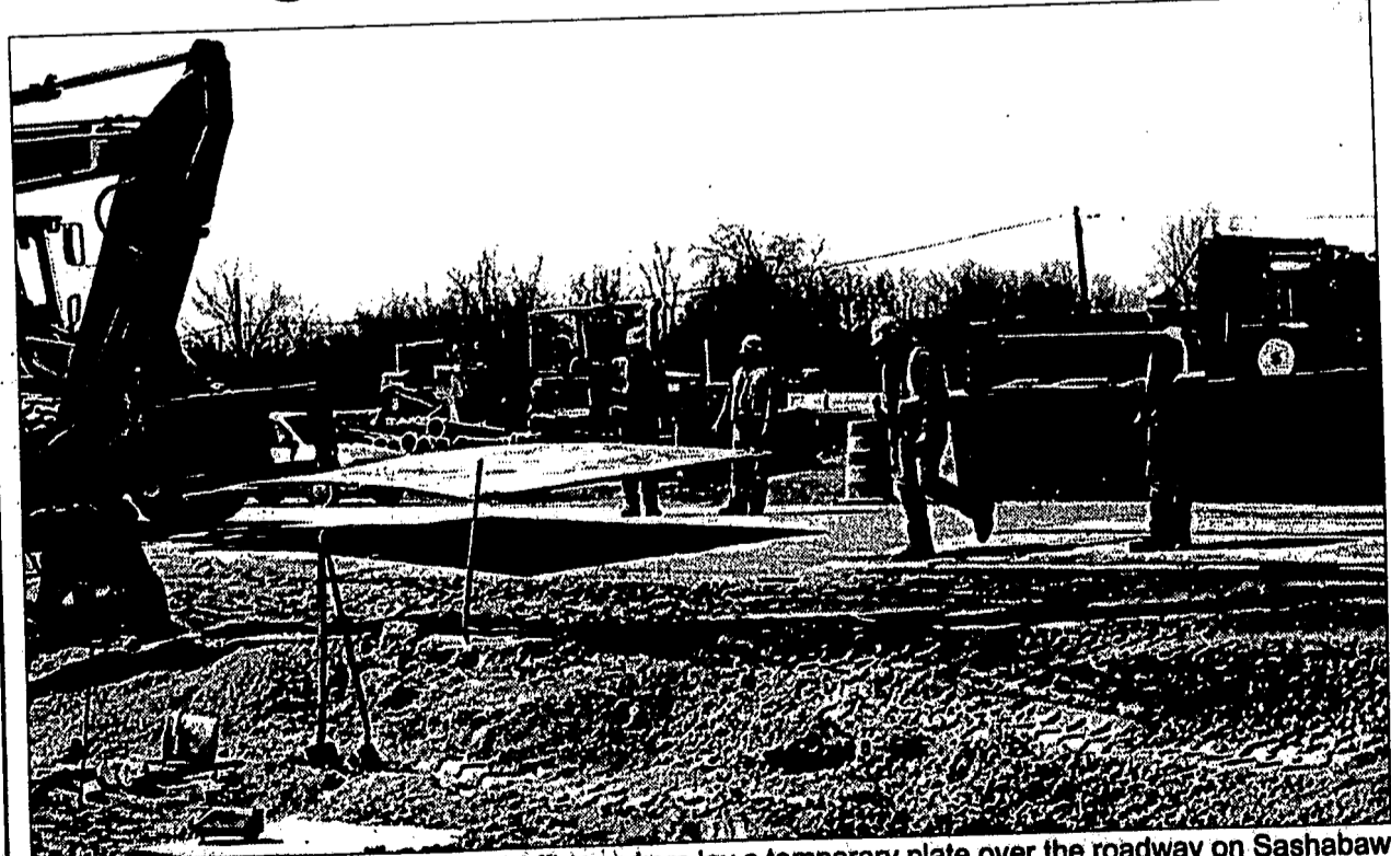
While reducing the road to one-way traffic, workers lay a temporary plate over the roadway on Sashabaw Road last week in one of the many places construction is ongoing between Waldon and Maybee roads. The project, which will result in a four-lane boulevard, will have intermittent lane closures throughout the spring and summer. Photo by Don Schelske
