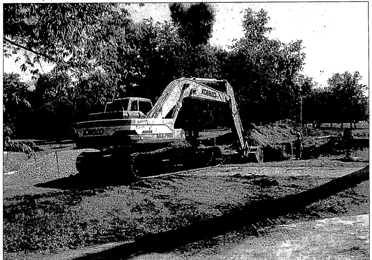
Excavation crews begin work in Clintonwood Park on the in-progress Spraypark on June 25. Al Doren of Independence Township helped coordinate the delivery of the crane for the work, which was brought in from Redford especially for the project. Photo by Alicia Dorset.
