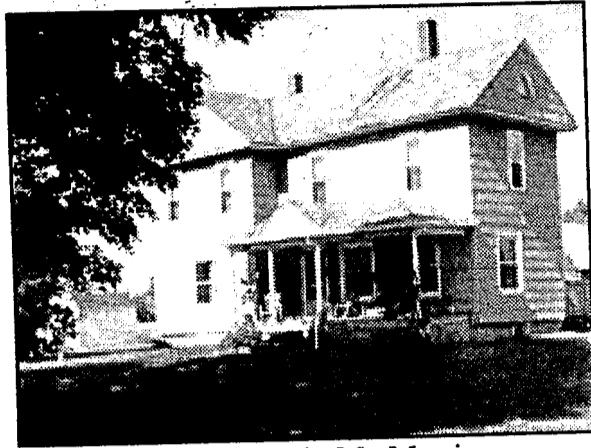
Genesee Road - Mt. Morris 5 Bedrooms - 2 Barns $149,900
