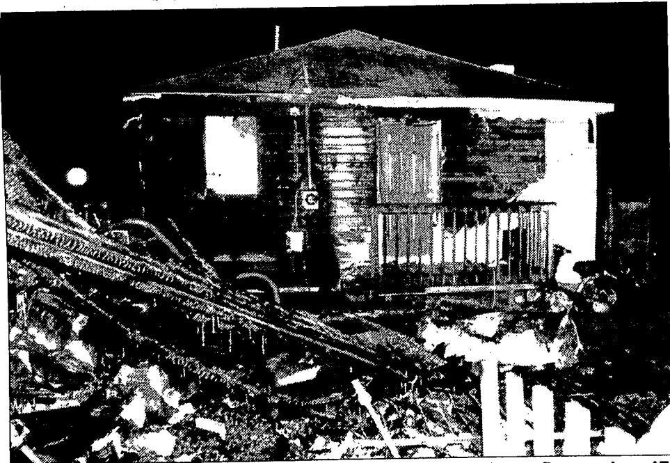
A Glenalda Drive home shows evidence of damage after a fire on Jan. 17. The house was damaged after fire destroyed a storage shed in the back yard. Photo provided by the Independence Township Fire Department
