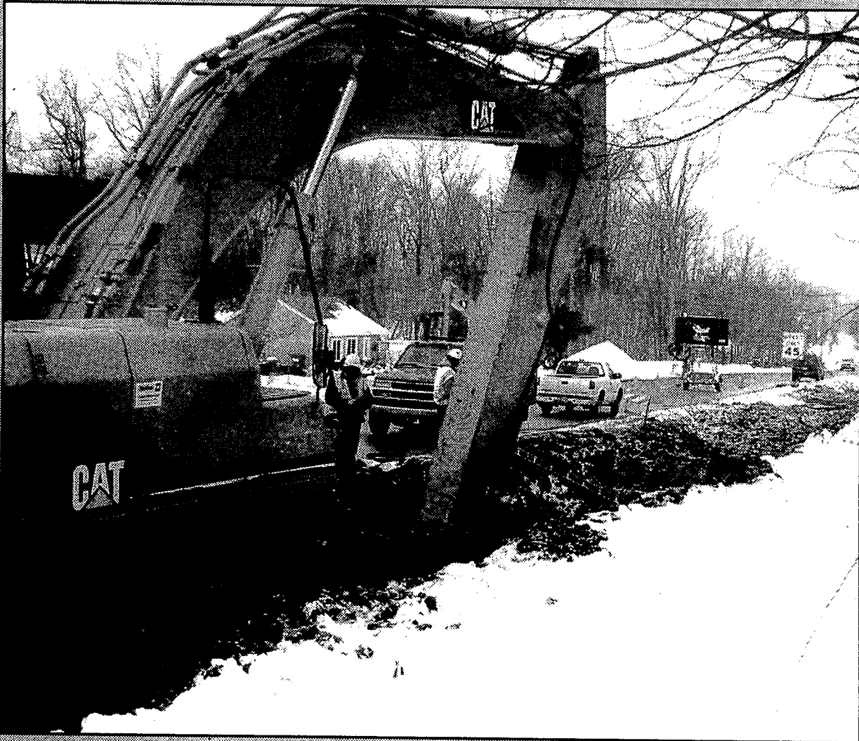
Construction workers brave the cold as they install storm drains along Clarkston Road just west of Sashabaw Road. Traffic was narrowed to one lane during the construction last week. While a major storm sewer project has yet to get underway, Independence Township DPW Director Linda Richardson said the current work is in relation to a new commercial building under construction at the southwest corner of Clarkston and Sashabaw roads. Photo by Don Schelske
