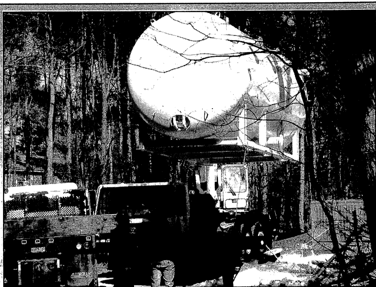
Workers balance a large water storage tank as a crane lays the equipment in place at a treatment well near the Deerwood Road area. Photo by Jenny Matteson
