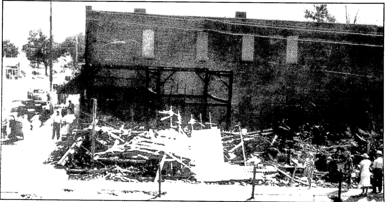
In 1939, the Clarkston Venetian Blind Company, located behind Rudy's Market, caught fire causing all three buildings to burn. The building pictured standing is now The Clarkston News office.
