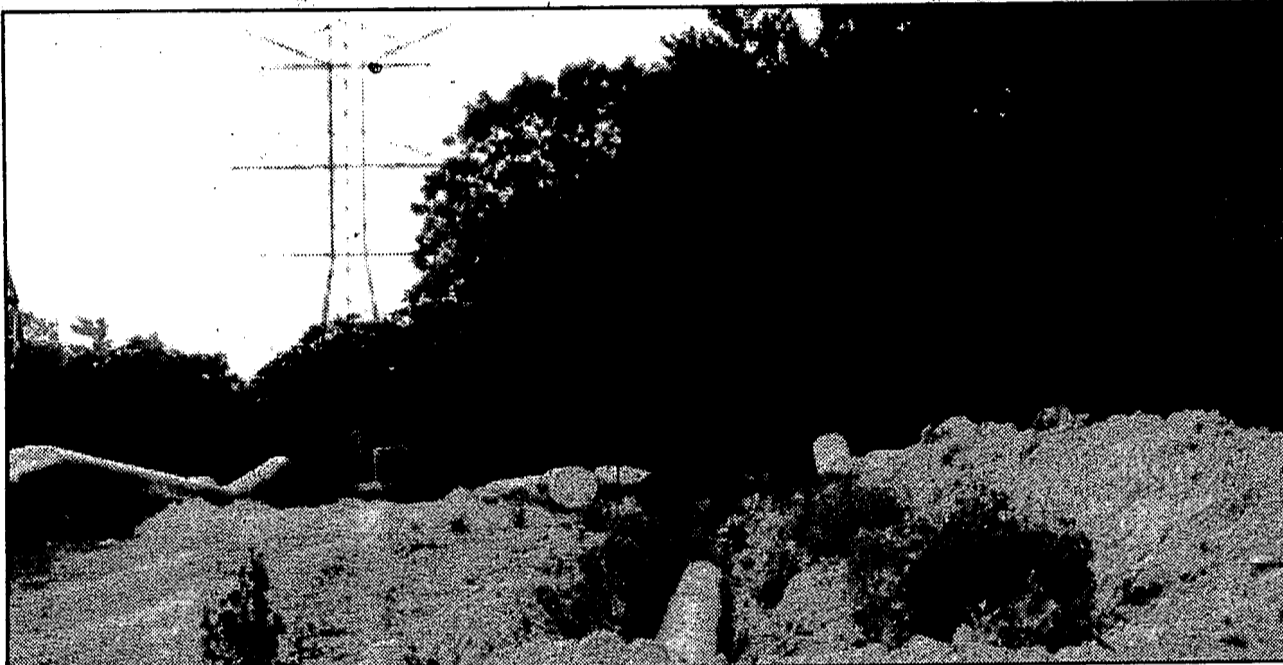
Consumers Power installing pipelines through Chestnut Hills subdivision. Photo by Heather Clement
