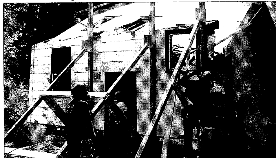
The training required building braces to stabilize the house.
