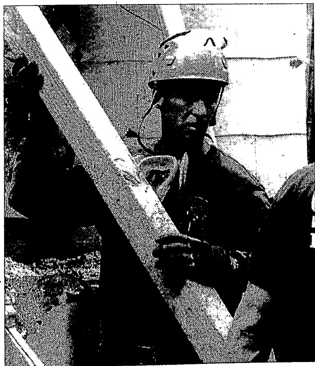
Bracing the collapsed structure was important to allow emergency personnel to safely work in the collapsed wooden structure.
