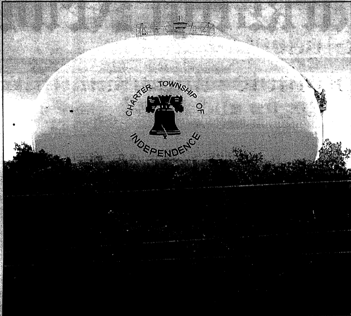
The watertower along I-75 in the industrial zone near Sashabaw Road sports a new Independence Township sign greeting drivers across the area. The watertower is brand new and part of the township's water system upgrades. Photo by Noah Purcell
