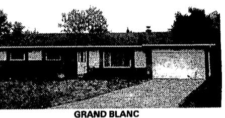
GRAND BLANC Cute brick ranch situated at the end of a cul-de-sac. 1300 sq. ft., 3 bedrooms, 1 full and 1 half bath. Living room, plus family room with gas fireplace. Newer vinyl windows. 2 car attached garage. Fenced backyard. Central air. Nice home! (5626M) $153,900
