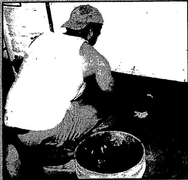
A worker with Midwest Waterproofing smooths the concrete on my newly repaired basement. Photo by Tom Matteson
