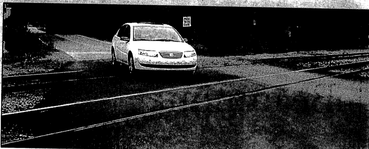
Drivers have a newly repaired crossing to drive over on Big Lake Road in Springfield Township. Photo by Paul Kampe
