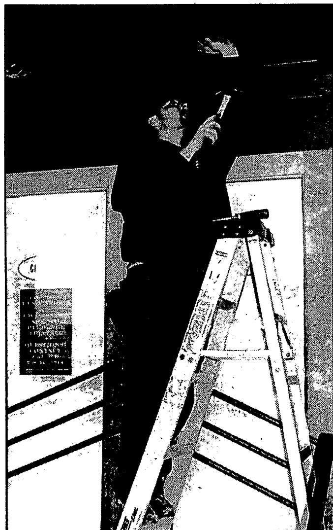
Robert Poe of Churchill Electric works on the lighting at the entrance of Clarkston Cafe. The remodeling work is nearing completion. Photo by Phil Custodio
