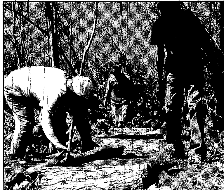
Volunteers began work on a corduroy bridge that will eventually allow access to the riverbank.
