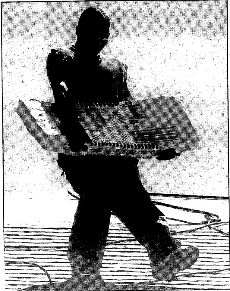
Ricky Chamelrain carries a pack of tiles across the roof.
