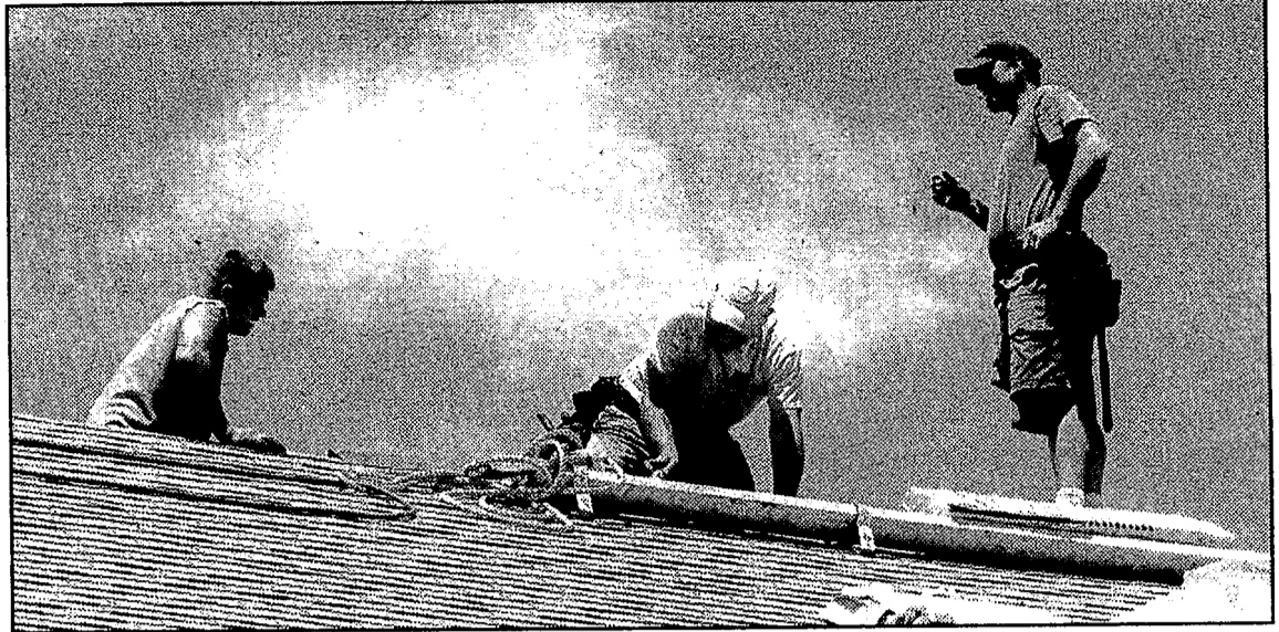
Workers Ricky Chamelrain, Dallas Oliver and Ed Lamielle lay new tiles.
