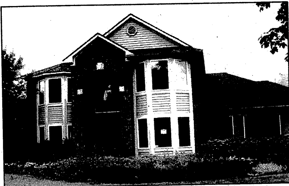
Above sits an abandoned house on Dixie Hwy. after foreclosure. At right is a common sign seen on foreclosed houses.
