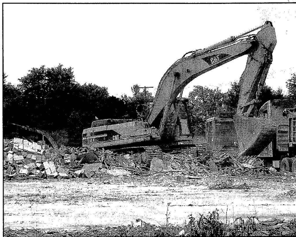
Workers scoop up debris from the former South Sashabaw Elementary School on Maybee Road. Photo by Phil Custodio
