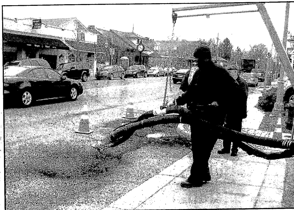
The first step was to fill in holes with alternating streams of liquid asphalt and gravel.
