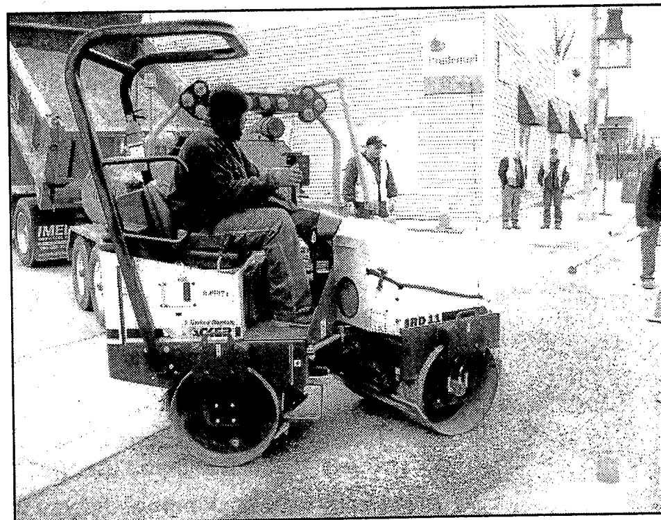
After the pothole is filled, it's compressed with rollers. Photos by Phil Custodio
