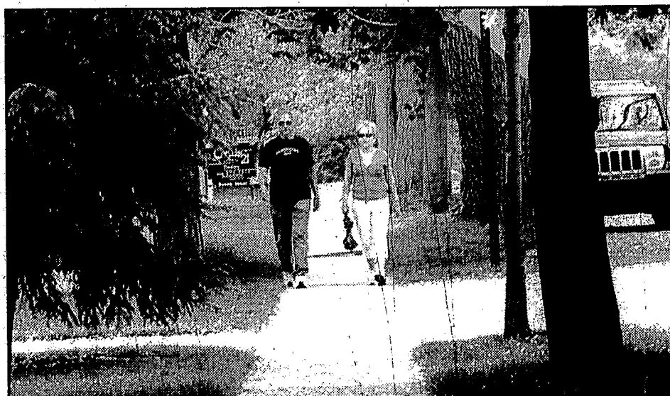
According to Clarkston City Council, sidewalks along Holcomb need repair. Photo by Trevor Keiser
