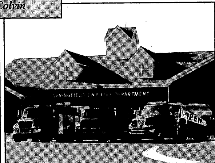
Firehouse renovations cost about $1.1 million and increased station no. 2's total area from 2,500 to nearly 13,000 square feet.
