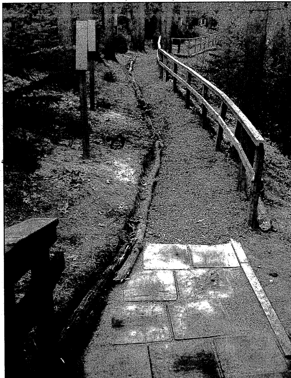
The finished trail, with new fence, mulching, and Stations of the Cross.
