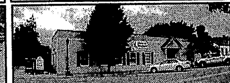
Ortonville Office for Lease. SO48 $500
