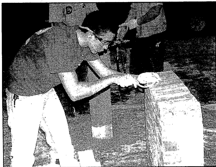
Ben Hunter of Oakland Technical Campus Northwest finishes the final touches on his wall.
