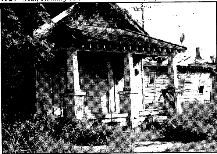
As time goes by, the condition of many homes grows worse as rot and decay set in.
