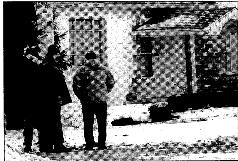
Clarkston City Manager Dennis Ritter, Councilman Jim Brueck, and resident Norm Cristea examine a sinkhole in Cristea's yard. Photo by Laura Colvish
