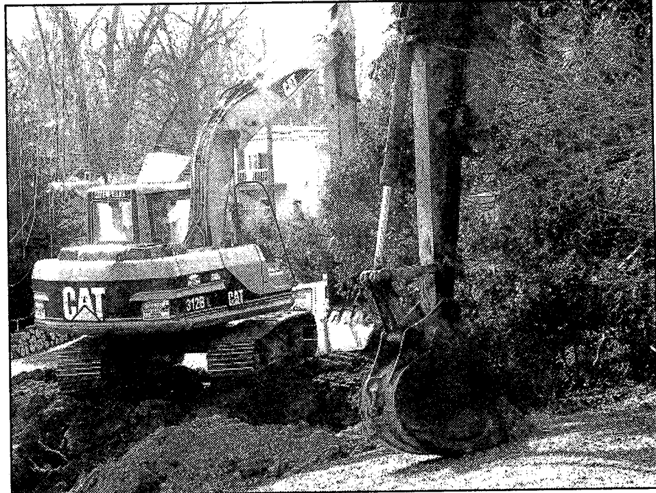
Construction equipment will soon be gone.
