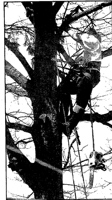
A Detroit Edison worker frees power lines from a fallen tree. Photo courtesy of Joyce Nienhuis
