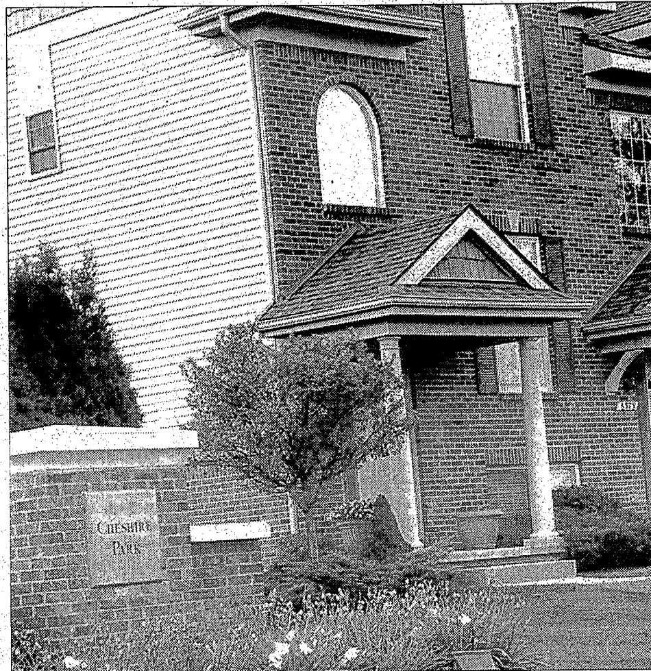
Cheshire Park sanitary sewers has been connected to the wrong pipe the past four years. Photo by Trevor Keiser.
