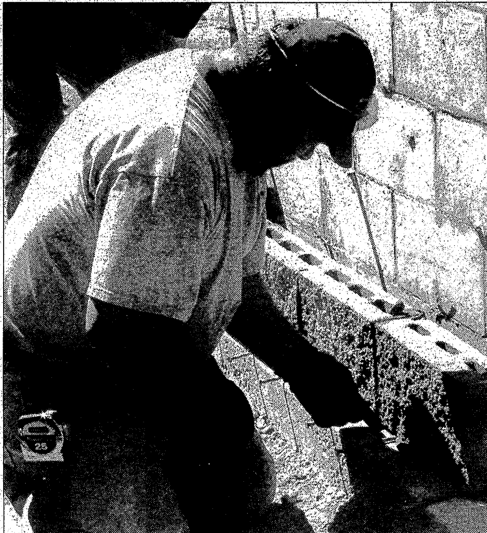
Tony Hool scrapes the excess mortar from the brick crevices.
