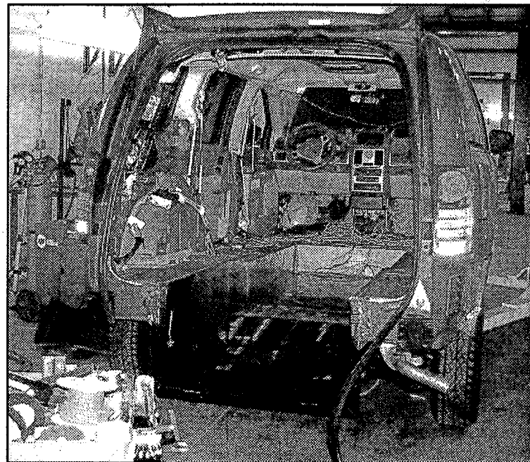
The conversion includes cutting the floor and rear frame of the minivan.
