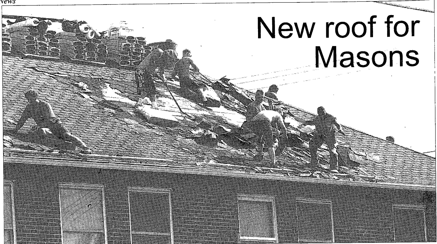
Workers strip four layers of shingles from the roof of Cedar Lodge 60 in downtown Clarkston. Photo by Phil Custodio
