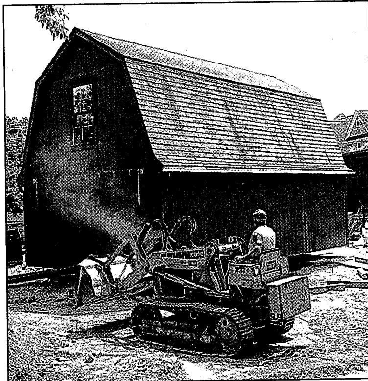
The structure will be converted into storage space.
