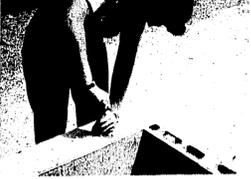
Screws pin the sill to wooden blocks
