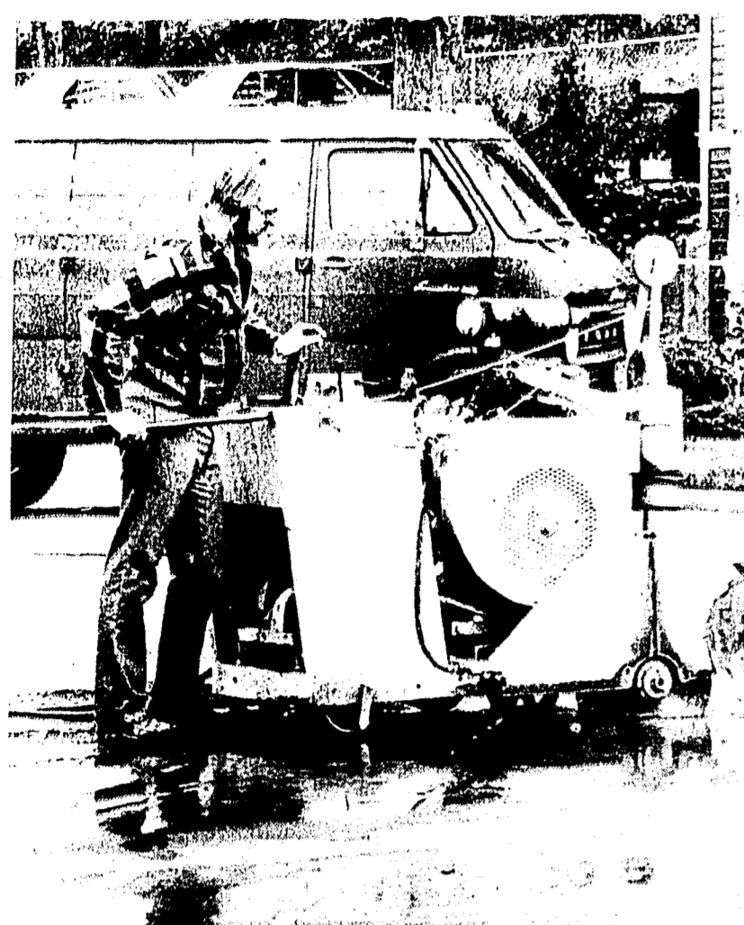
WHEN THE CONTRACTOR required a cut through the pavement on Center Street in Northville so that giant new pipe could be installed for the Randolph Drain he called on a local firm — International Concrete Drilling & Sawing Company—to do the job. The company is operated by Marian Szecepanski and his son, Victor (above). The parent company, International Diamond Tool Company, 21141 Novi Road, is one of the nation's leading diamond tool research and development firms.
