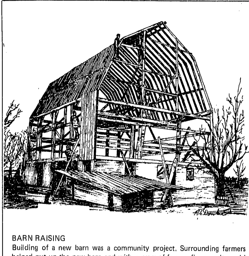
BARN RAISING Building of a new barn was a community project. Surrounding farmers helped put up the new barn and with a crew of four or five men it would probably take about a month to complete. This raising took place in 1907; it is the barn on Mr. and Mrs. Foster's farm on Pontiac Trail.
