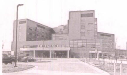
Providence Park Hospital is part of St. John Providence, the largest provider of inpatient care in southeast Michigan.
