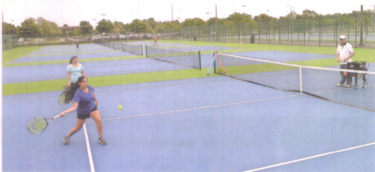
After undergoing a summer-long renovation, the Novi High School and Civic Center tennis courts are back in action. The courts received new fencing, walkways, nets and court surfaces. Here, sisters Christina, 14, and Serena Shina, 11 take a lesson from Nick Falice.
