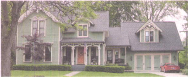
This Randolph Street home is on the Sept. 26 tour.
