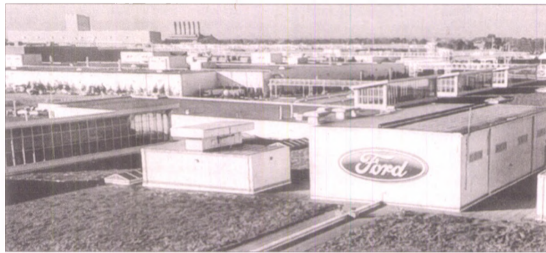
The "living roof" atop the Ford Rouge Center in Dearborn has become an iconic symbol of the company's sustainability ethos.
