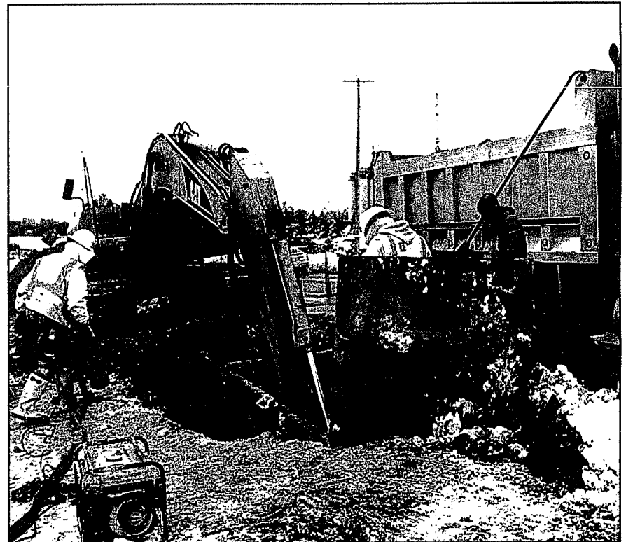
Independence Township DPW contractors work to repair a leaking 12 inch water main on White Lake Road near the railroad tracks. Photos by Andrea Beaudoin
