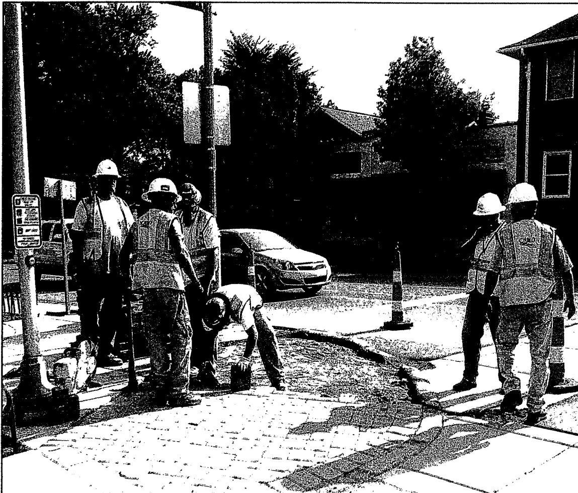
Crews from Carlo Excavating removed brick pavers from the sidewalk at Main and Washington streets on Monday. The bricks were taken to the City of the Village of Clarkston for reuse in community projects. Photo by Andrea Beaudoin
