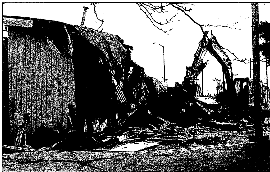
Workers demolish a closed gas station on M-15. Photo by Andrea Beaudoin
