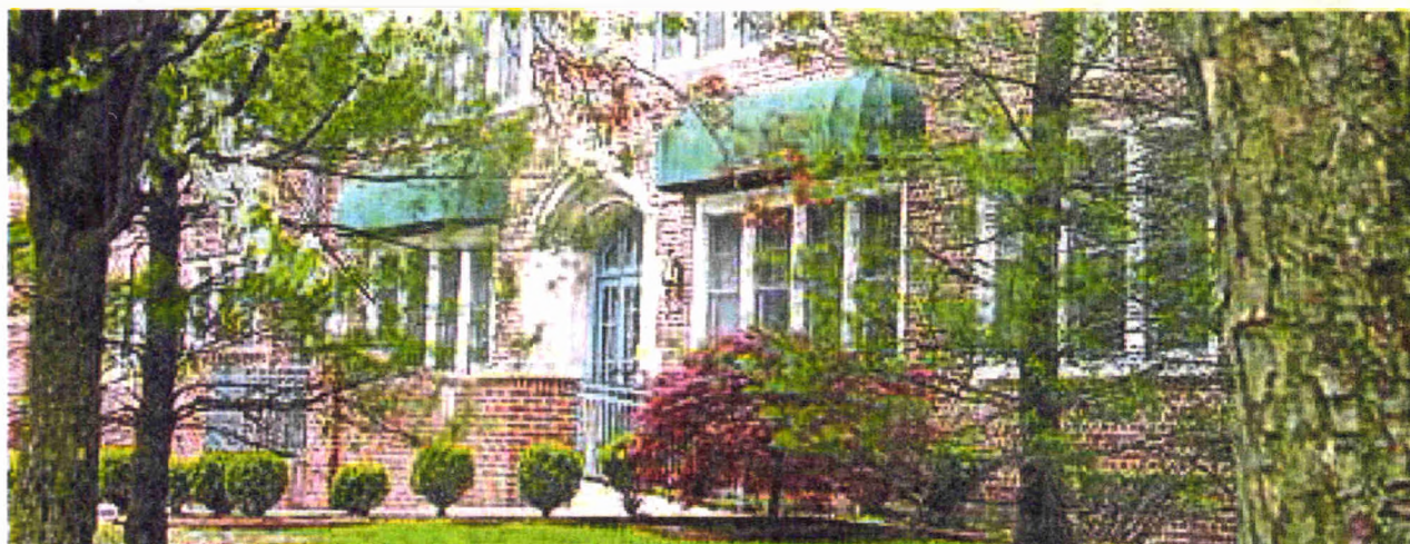
This Albert Kahn building in Farmington Hills, now part of Botsford Commons, is the former home of the Sister Kenny Hospital, where children with polio were treated in the 1920s.
